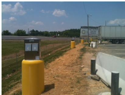
Southern Pride Truck Plaza, located at Exit 16 on I-24 in Paducah, now has new technology which saves money, reduces noise, and cuts down on emissions. The truckstop now has 24 parking spaces with plug-in power pedestals. Shorepower Technologies developed the plug-in power pedestals which provide access to power sources, at a rate of \$1 per hour.
