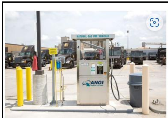
CNG Fuel Station
